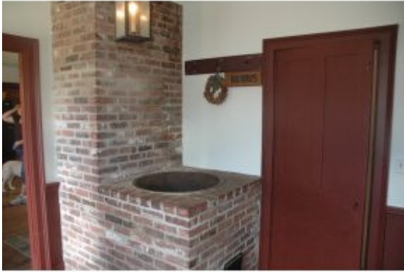
Cistern with its own flue
